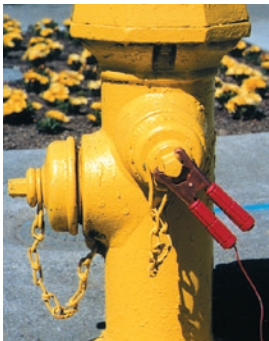
Clean off rust and old paint for a good connection.
